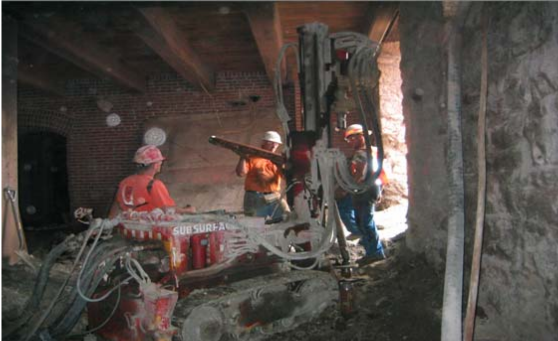
Cupples Station Building 1 – Downtown St. Louis, MO – Building Retrofit with Micropile
