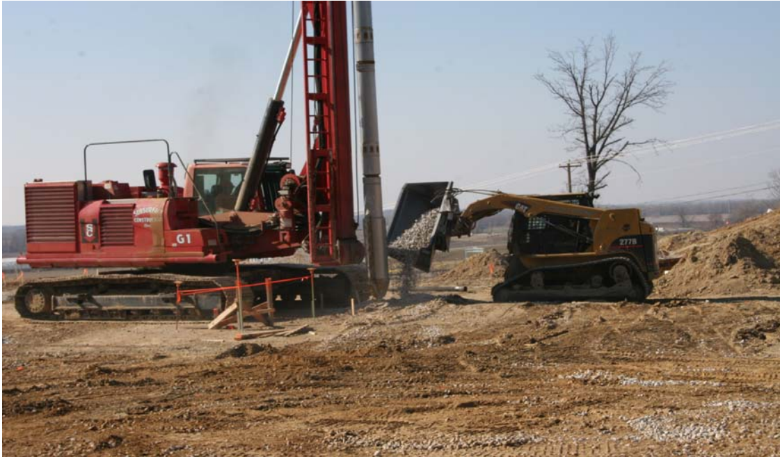
Stratacaster Rig Installing Stone Columns
