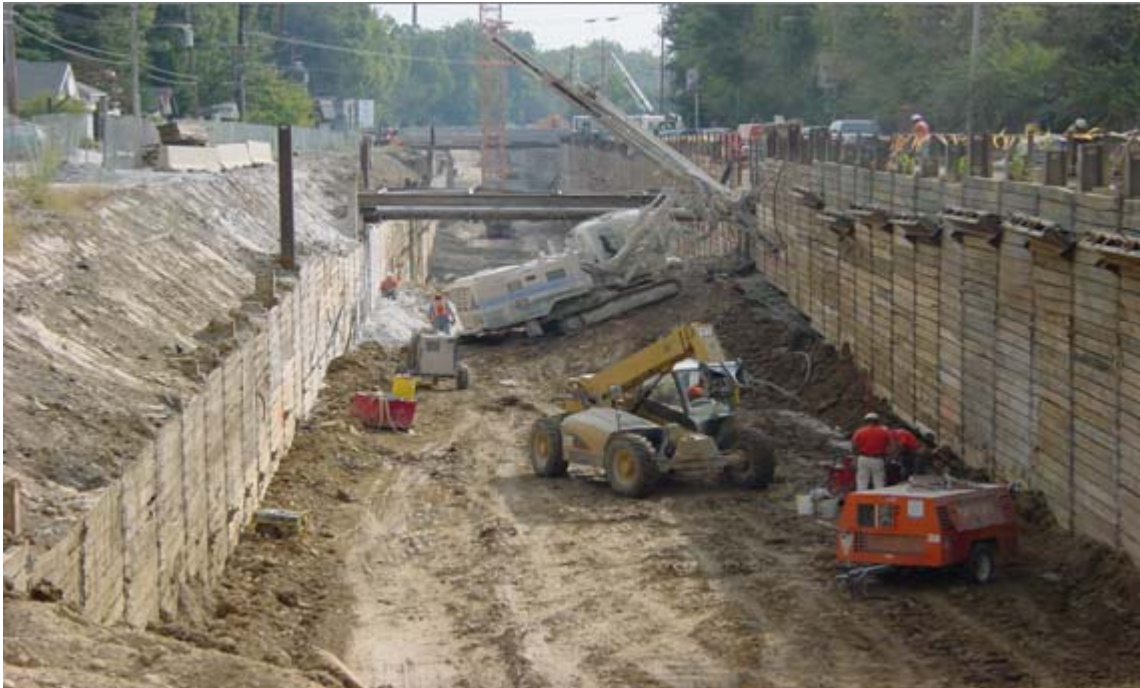
Furukawa Rig Installing Tiebacks
