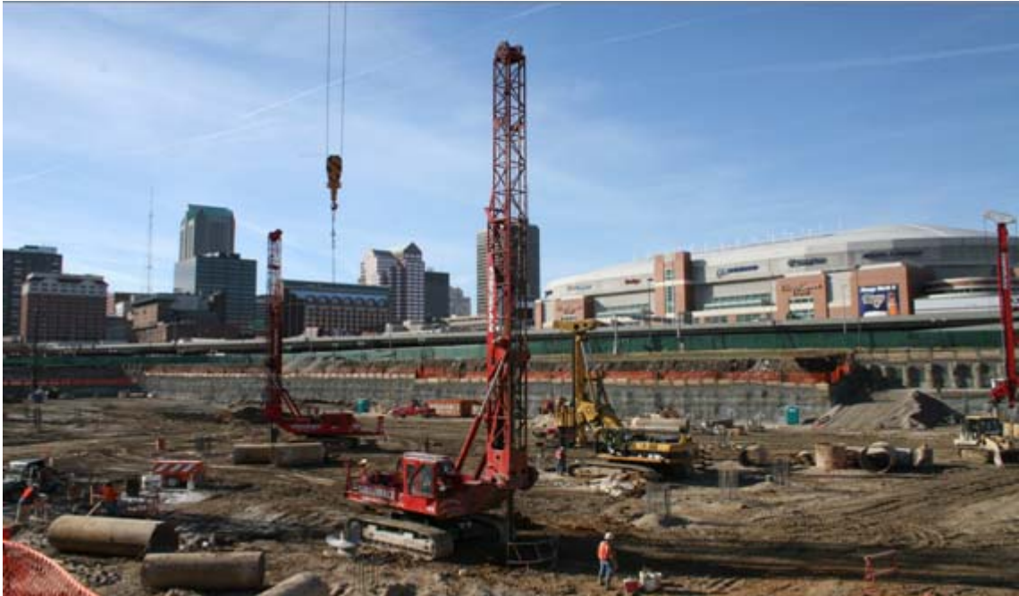
Pinnacle Casino, St. Louis, MO – Drilled Shafts and Earth Retention
