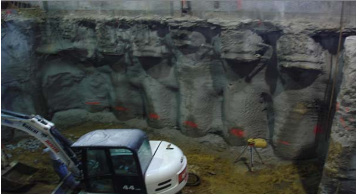
Underpinning Existing Exterior Wall / Excavation Shoring
