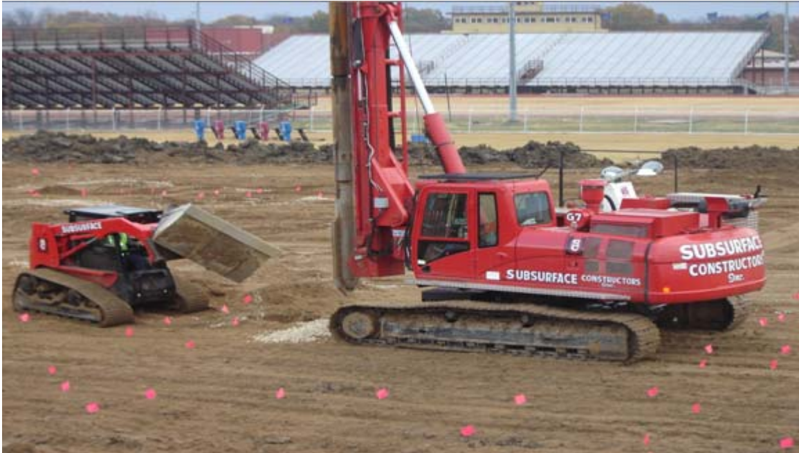
West Memphis High School Auditorium, Vibro Stone Columns
