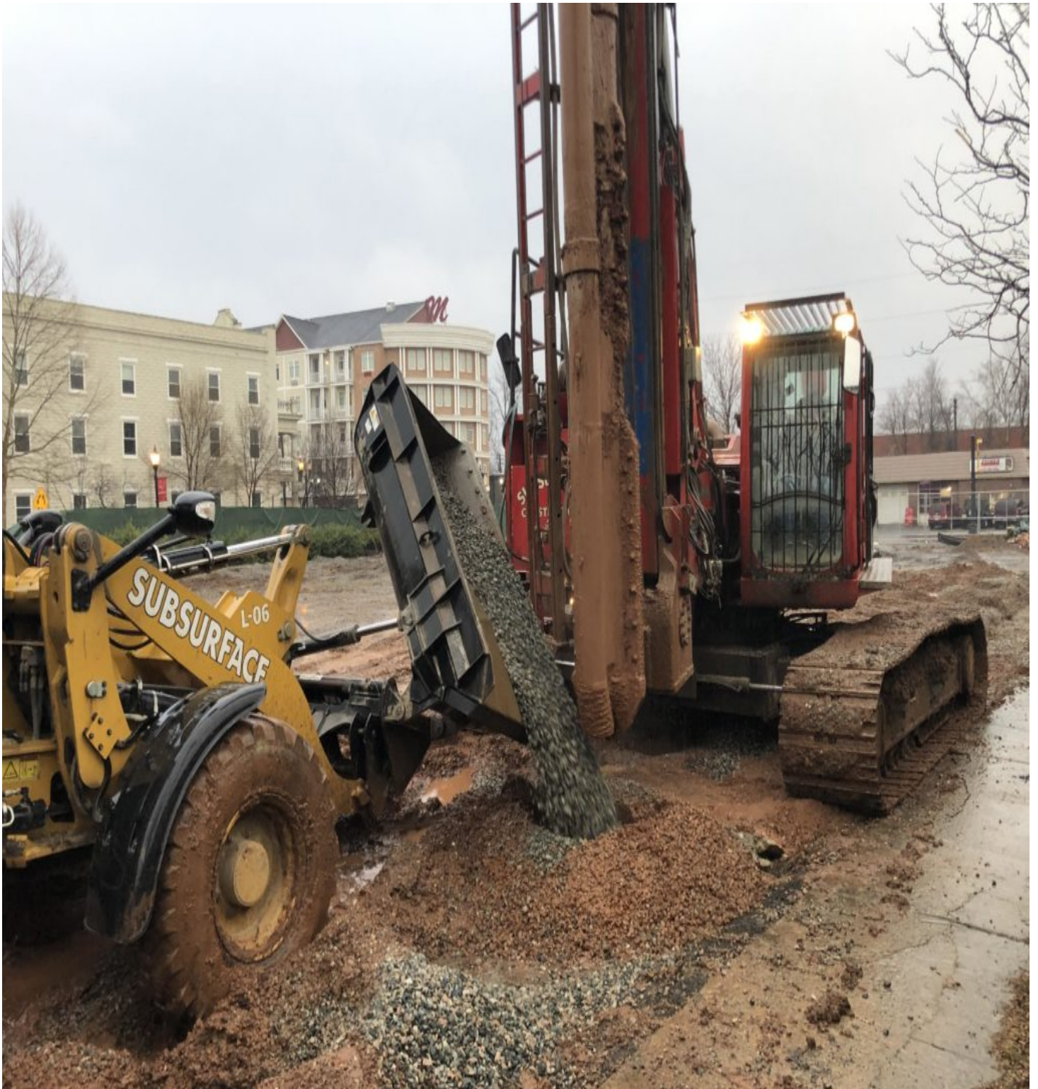
Aggregate piers for ground improvement on seven-story development
