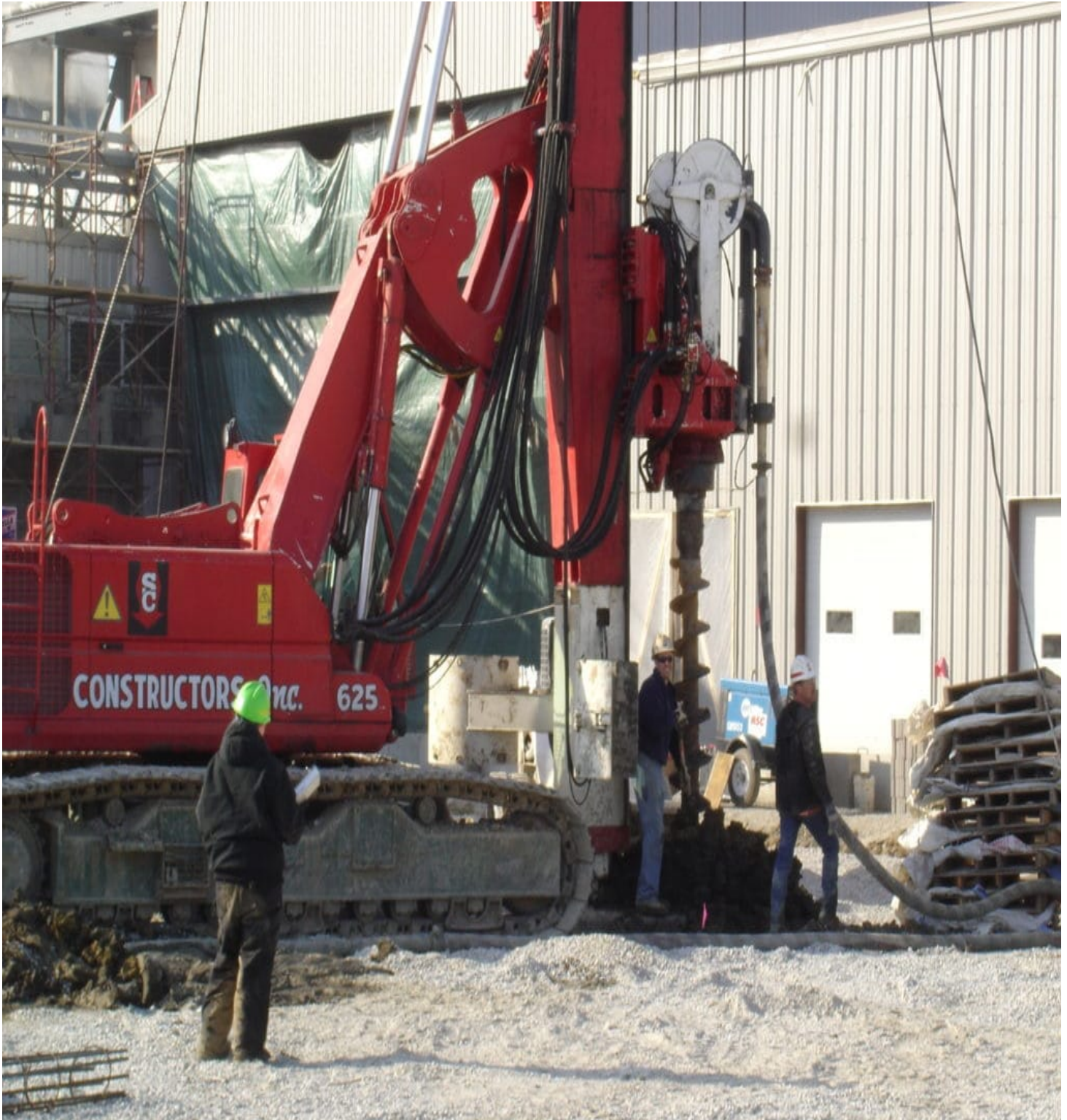
Augercast piles for Proctor & Gamble building addition
